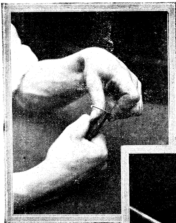
Fig. 4.—Bending square section wire.
